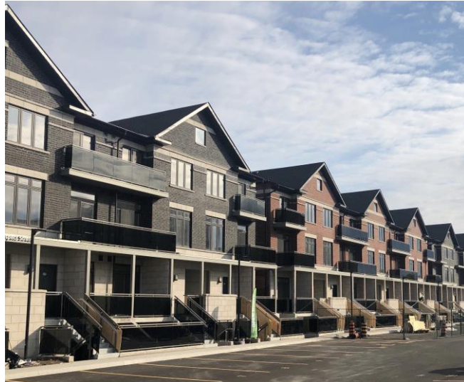
2051-2073 Prospect Street, Burlington ON
