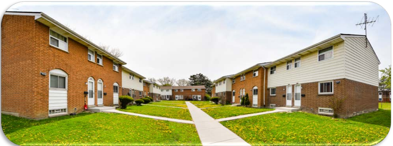
2602 – 2682 Sycamore Drive & 7750 – 7738 Hawthorne Drive
